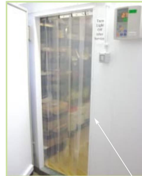
*A PVC Curtain to reduce temperature loss when opening door*
