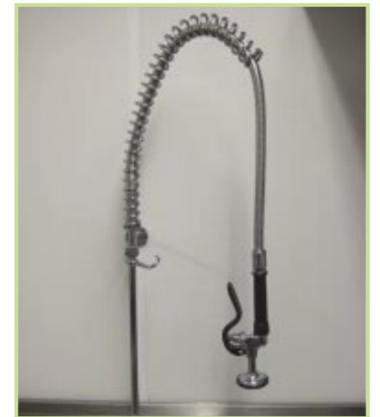
In your kitchen install low flow trigger operated spray taps and hoses.
