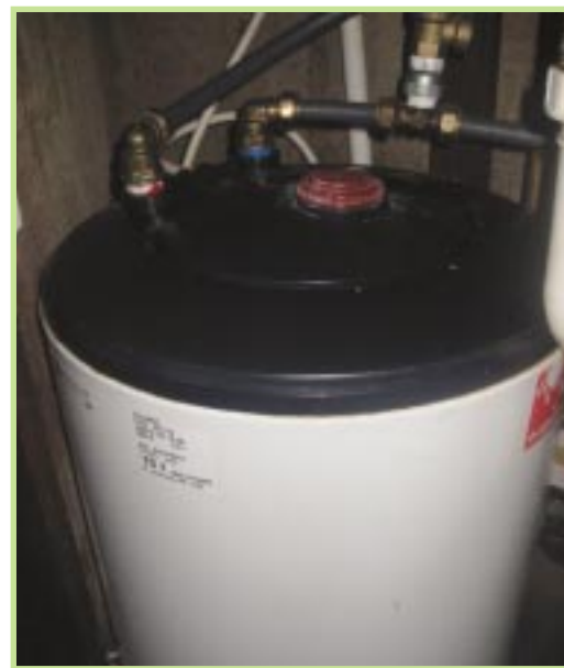
Under counter hot water heaters – an efficient way to provide hot water
