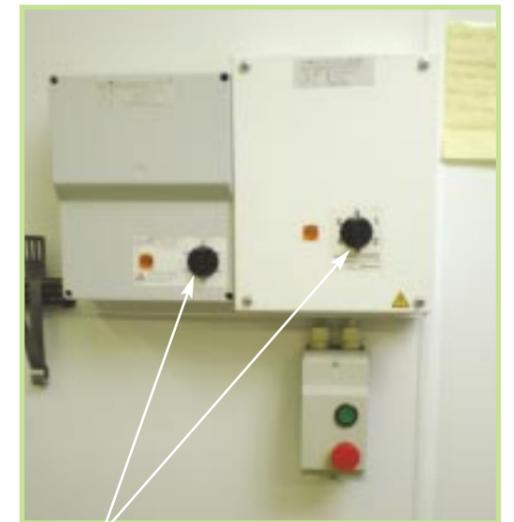
*Variable speed drives can reduce energy consumption for extractor fans*
