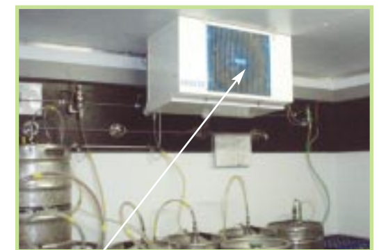
Keep evaporator fins clean
