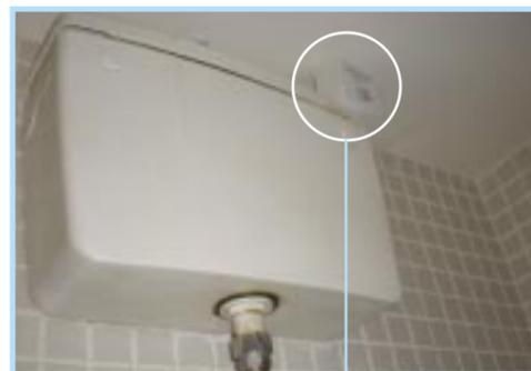
Motion sensor which has been retrofitted to urinals to conserve water and save
