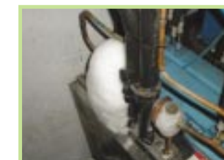
A poorly maintained beer chilling system. Ice build up indicates poorly insulated pipe-work on refrigeration.
